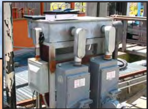
200A MaxGard interlocks in parallel
